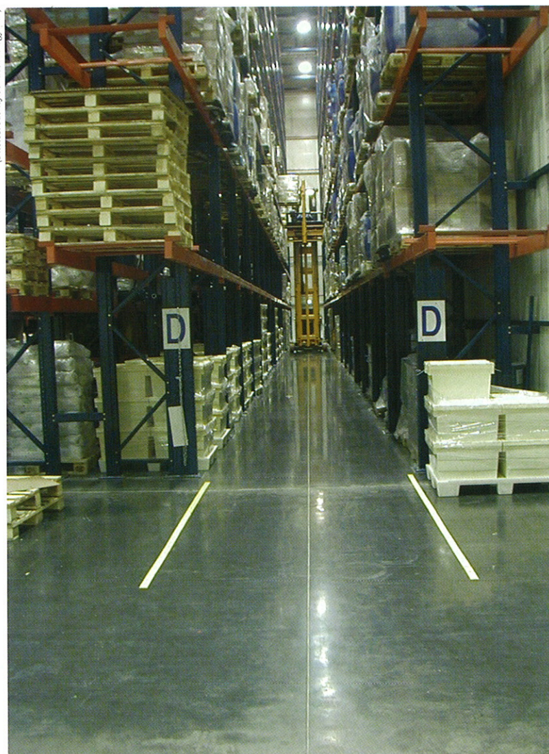
Figure 1: Completed Superflat floor.
